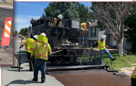
Cap Seal Resurfacing
