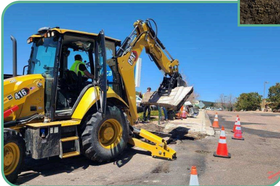
Gaining Access and Shoring For Valve Repair at Monument Plaza
