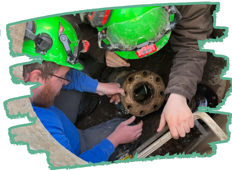
Replacing a Meter
