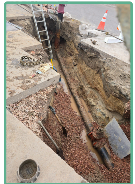
Replacing a Valve at Monument Plaza
