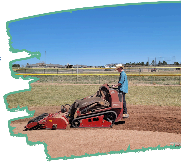
Resurfacing Santa Fe Ballfields
