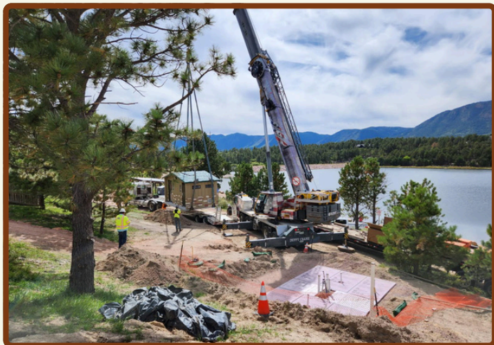
INSTALLING NEW BATHROOMS AT MONUMENT LAKE
