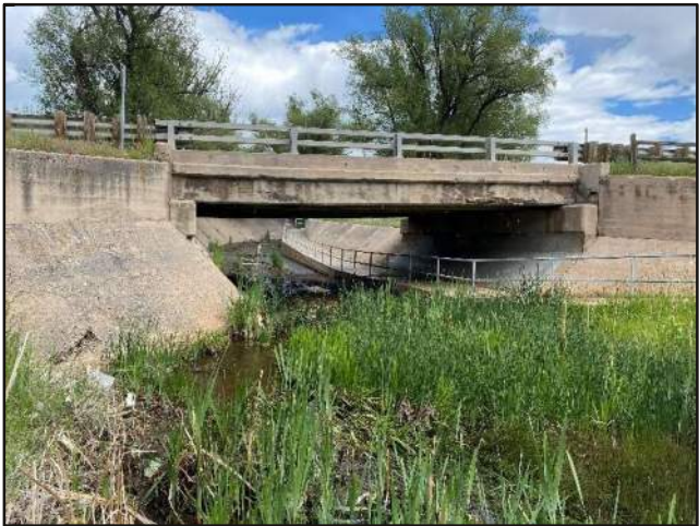
Photo 3: C06-struct01. Crystal Creek at Highway 105 looking north.
