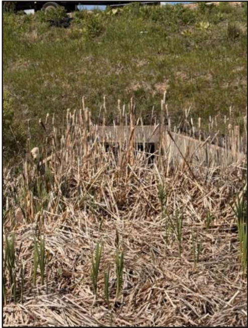
Photo 26: T01A-struct01. Cattail/reed overgrowth. Teachout Creek at Access Road/I25 crossing.
