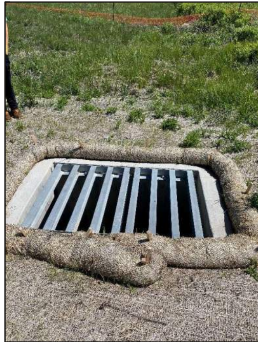
Photo 31: Upstream grate flush with grade. Water will overtop Bowstring Road.
