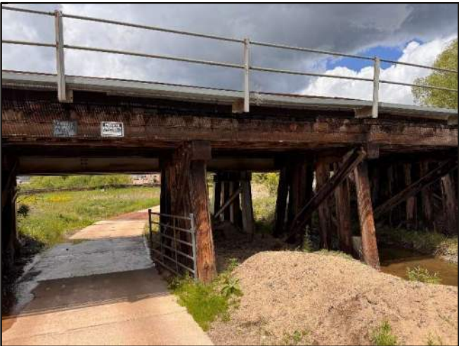
Photo 28: T03-struct01. Teachout Creek at Union Pacific Railroad crossing (north). Upstream pond held by beaver dam(s).
