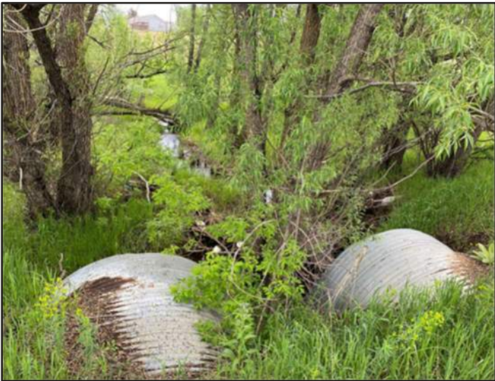
Photo 5: C05-struct01. Crystal Creek at Washington Street.
