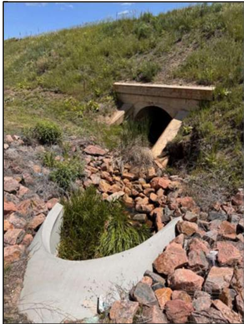
Photo 25: T01-struct02 (top) and T01-struct03 (bottom). Teachout Creek, between New Santa Fe Trail (top) and Old Denver Road (bottom).
