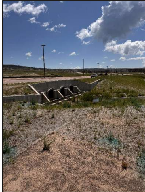
Photo 30: Teachout Creek NE of Jackson Creek Parkway, energy dissipation downstream of detention facility.
