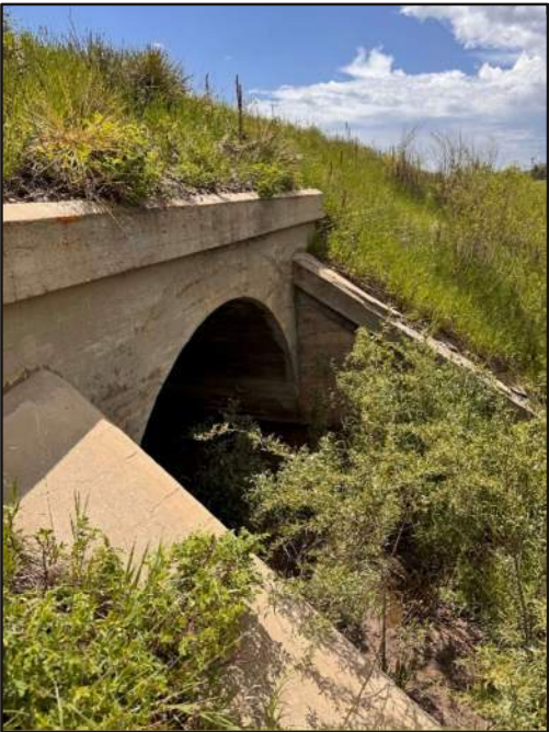
Photo 29: T04-struct03. Teachout Creek north branch at New Santa Fe Regional Trail.
