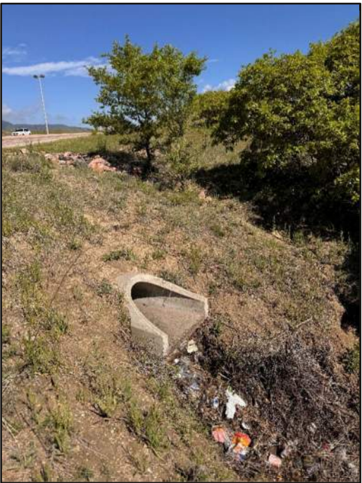
Photo 19: Jackson Creek Parkway outfall to Jackson Creek.
