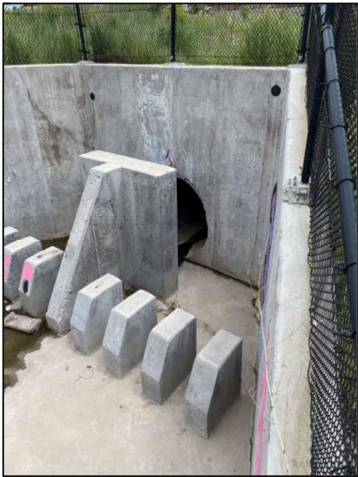
Photo 22: Energy dissipation at culvert outlet upstream of Monument Lake.
