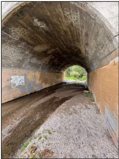
Photo 7: D03-struct01. Dirty Woman Creek at Union Pacific Railroad. Large bridge/tunnel structure.
