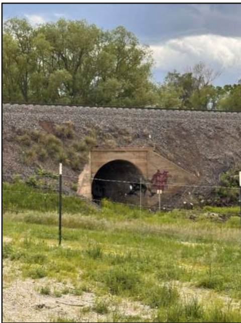
Photo 4: C03-struct01. Crystal Creek at Union Pacific Railroad.
