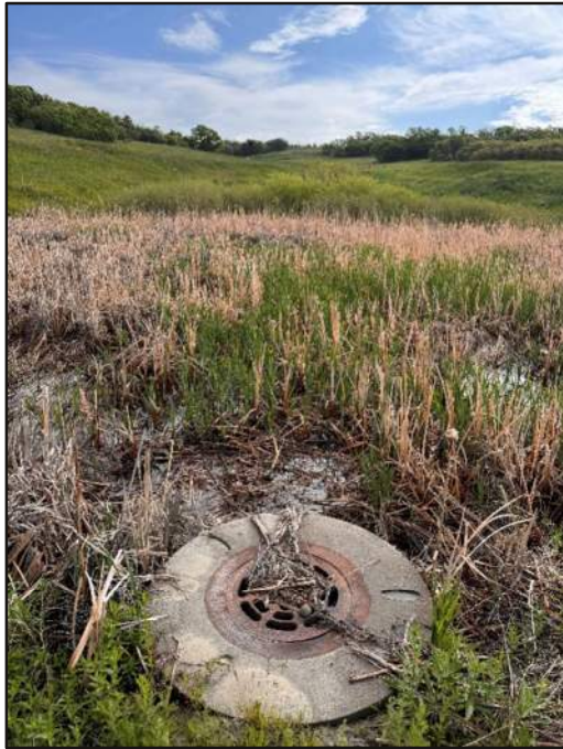
Photo 12: Overflow structure for detention basin on Jackson Creek upstream of Leather Chaps Drive.
